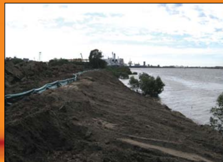
Preliminary earthworks between Cormorant Road and the river
